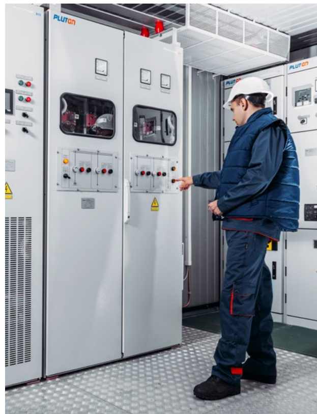
▲ Negative busbar switchgear
